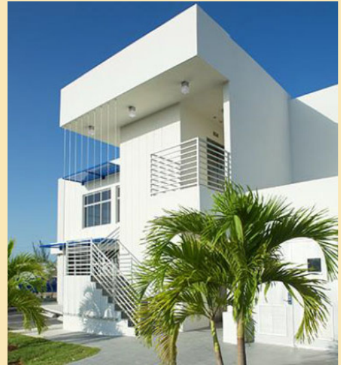
SWP's secure storage facility George Town, Grand Cayman
